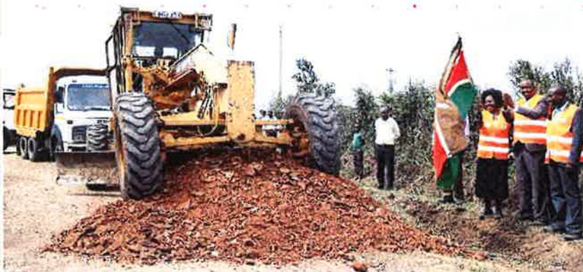
Kamongil-Kamosiro-Kaboson road, under construction
