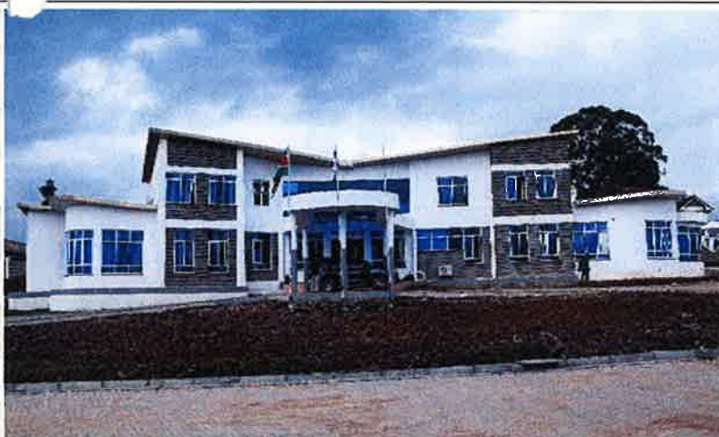
Completed Administration block
