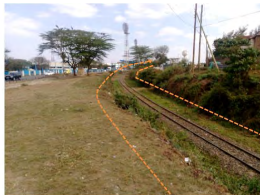
Behind the Nyayo Stadium. Enough space to accommodate dual lanes for BRT. Note that there is one round trip on KRC.
