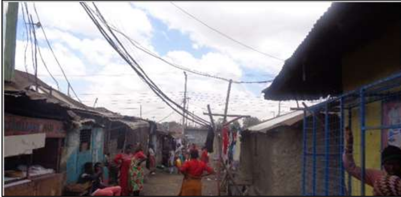
Figure 81: Unconventional Electrical Installations in Majengo
