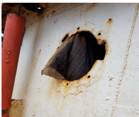
Porthole cover holding down bolts and nuts missing affecting watertight integrity.
